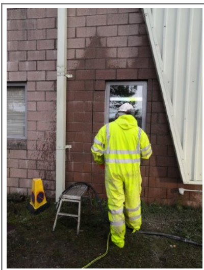
Diamond cutting the wall
